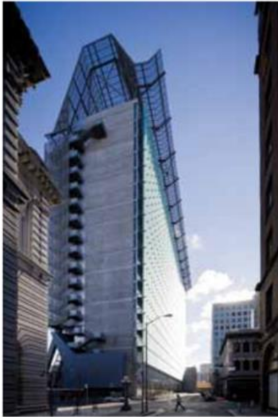
Figure 2. Type 316 perforated screens on the San Francisco Federal Building helped eliminate air-conditioning in 70% of the building's occupied spaces.
