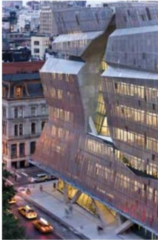
Figure 3. Perforated Type 304 screens give 41 Cooper Square a sculptural appearance while reducing the building's energy consumption. © Iwan Baan Studio
